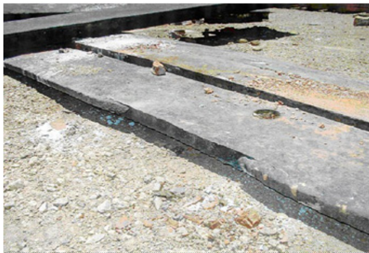
Figure 1: Corroded copper block cooler in sulphuric/ sulphurous acid condensing environment
